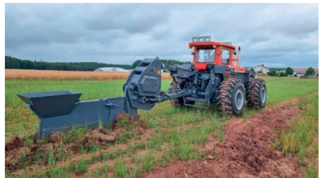
Plowing with a sand backfilling chute
