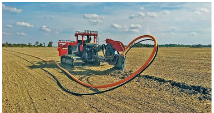
Plowing in of a gas pipeline HD-PE OD 110 and cable protection pipe OD 50
